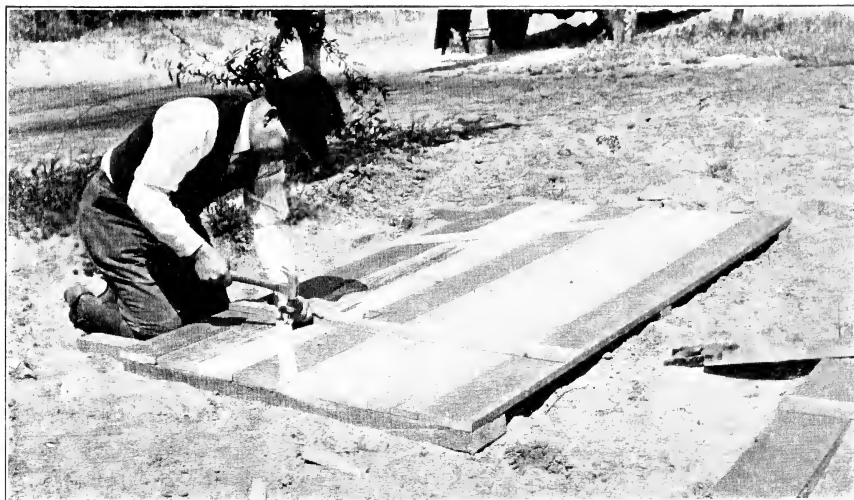
Fig. 8—Nail the 1×2-inch baffle cleats firmly in position after trimming the side-wall sheathing.
